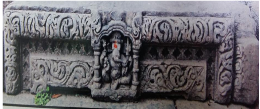
Pl.4. Lintel of a ruined Temple in complex.
