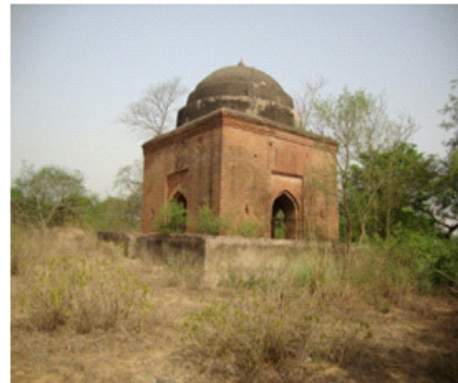
Plate 2: Another General View of Gumbad Imadul Mulk.
